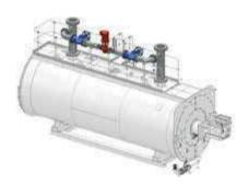
To maintain the minimum return temperature and the maximum flow/return  $\Delta T$  within the allowed limits, a recirculation system is installed between the flow and return connections which recirculates a suitable water flow rate in order to raise the return temperature before it goes into the boiler.
